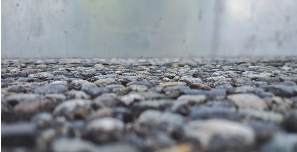
Fig. 14. Transverse regularity of the existing pavement (detail c)
