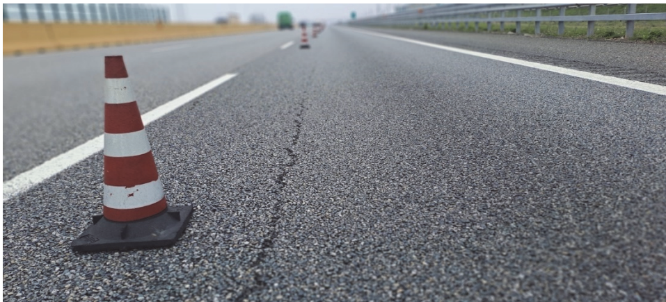
Fig. 12. Existing pavement monitoring (detail a)
