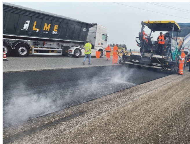
Fig. 3. Paving stage of GPC modified AC
