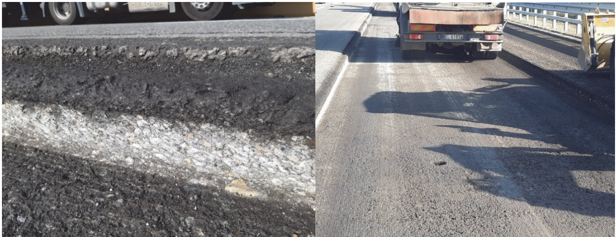
Fig. 2. Exiting pavement detail after the milling operation
