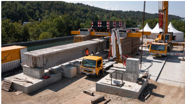
Fig.3. The testing layout is depicted in (a), with measurements in centimeters. (b) provides a general view of the testing area.
